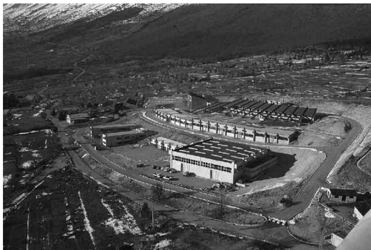
Figure 2. The LNGS outside facilities.
